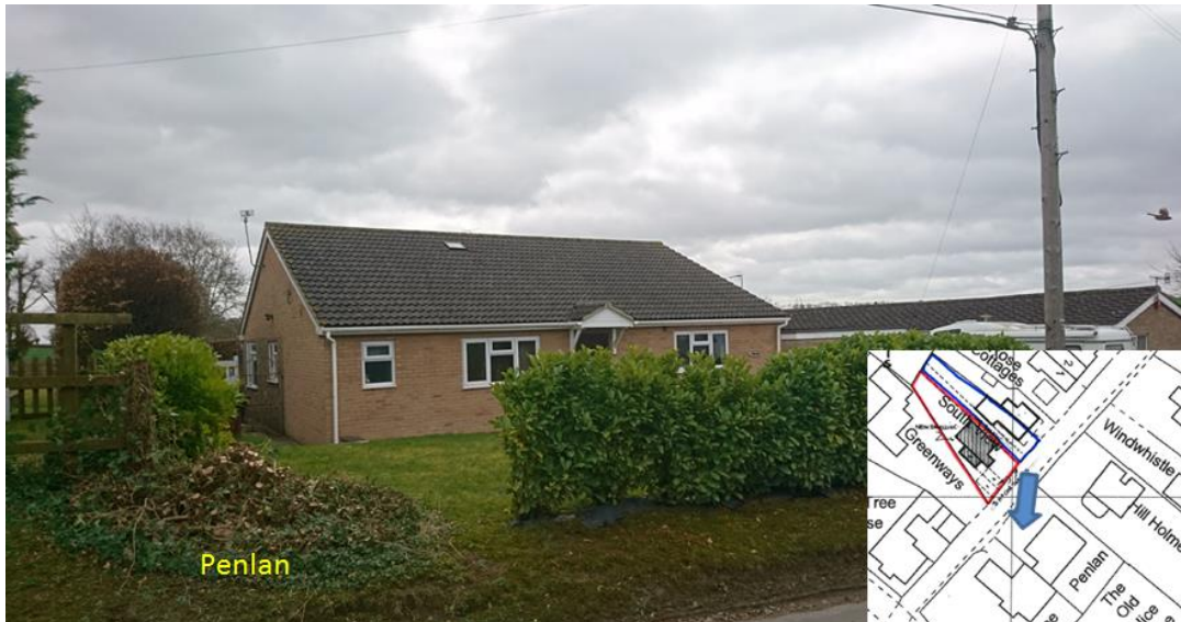
Front elevation of Penlan from Nett Road
